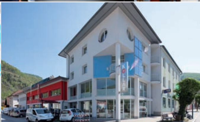
Kollar premises in Lilienfeld (Lower Austria)
