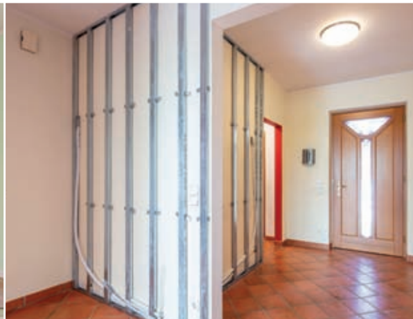
Installation of the U- and C-profiles in the entrance area
